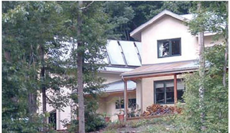
sustainable living. She used Hebel AAC blocks and panels for all of the walls and flooring throughout her 4,000 square foot house and saw immediate energy savings. Hebel AAC's thermal mass, coupled with solar panels and a wood stove, resulted in only \$100 in gas consumption during the first year she lived in the house. "Even when we lose power, the house will stay warm for two or three days," Dodson said.
