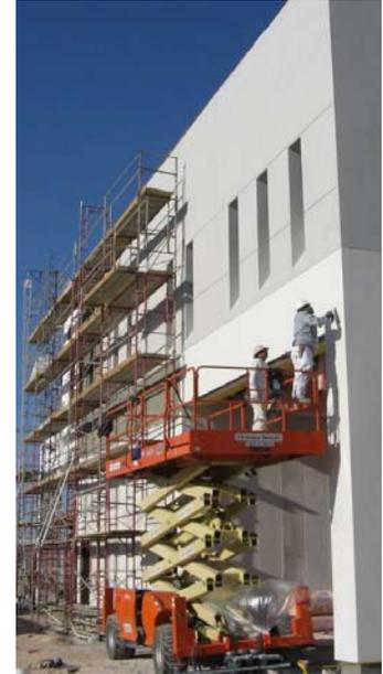
Figure 4.11: Applying coating to exterior AAC panels
