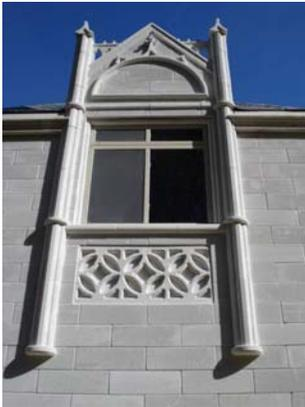
**Figure 4.3: Window trimmed with AAC**
