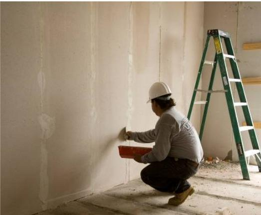
Figure 4.13: Filling AAC wall panels for a smooth surface
