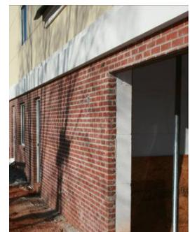
Figure 4.12: AAC with brick façade
