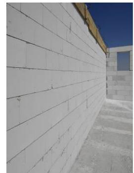
Figure 4.15: Interior AAC walls
