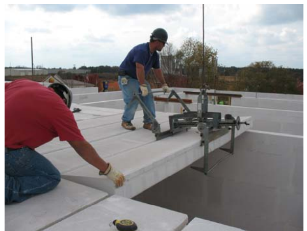
Figure 5B.5: Before placing the panel on the supports, clear safety bar from adjacent panel
