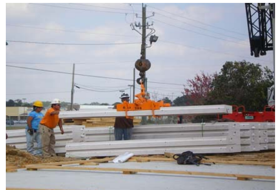
Figure 5B. 5: Placing the lifting gear at the center of panel
